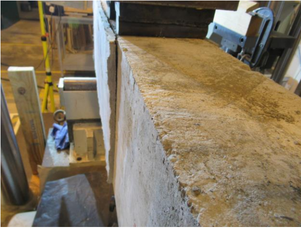
Figure 10: Debonding of SHCC at beam mid-span
