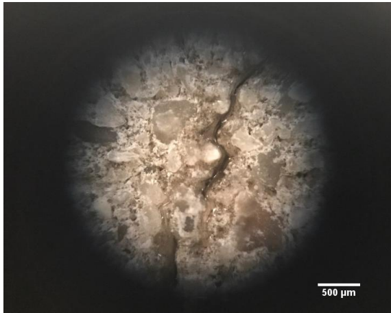
Figure 8: Filling of the crack by the sodium silicate (lateral face of the specimen).
