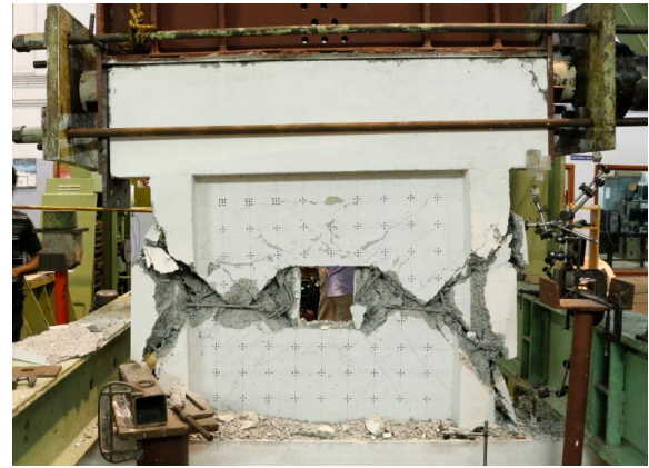
Figure 13: Crack pattern at Failure Load in SW-1.0-CW-IS
