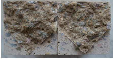
Figure 8: Damaged specimen with chevron notch.
