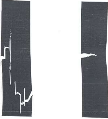
Figure 1: Crack development in fiber reinforced concrete (left) and in plain concrete (right).
