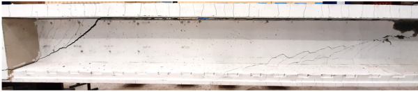
Figure 3: Crack pattern at the end of the experimental test taken from [14]
