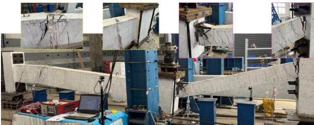
Figure 5: Crack pattern and failure mode of USRC.
