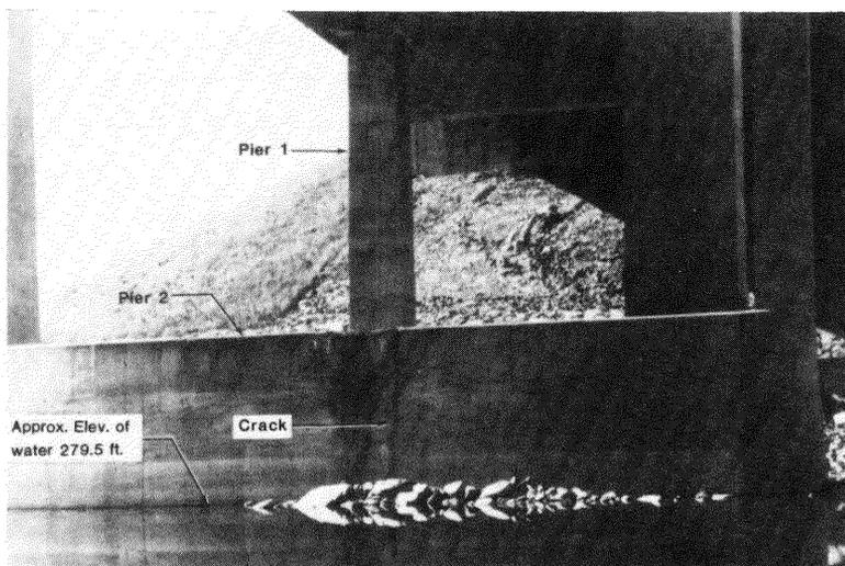
Fig. 7 Crack originating from top of plinth, soon after start of service. From Wiss87.
