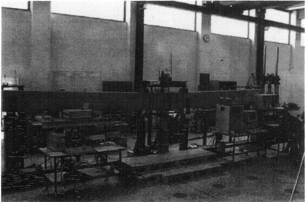
Fig. 1. Photo of the large beam. The data acquisition equipment (to the left) and the servo control (to the right) can be seen.
