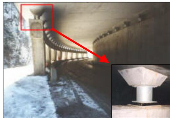
Figure 3. Photography of the new rock shed system - gallery "les Essariaux" - and a fuse support
