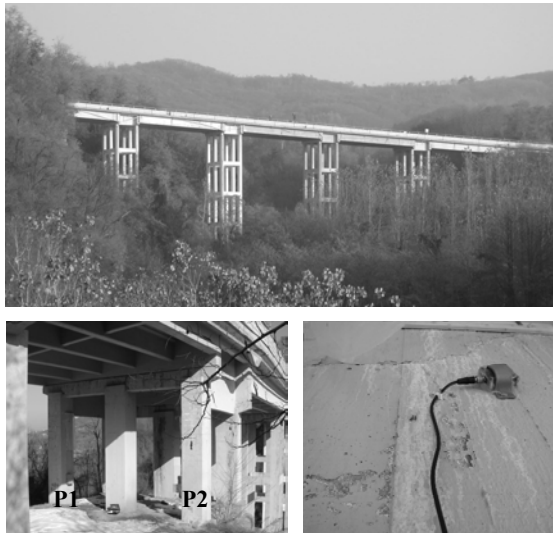
Figure 11. The viaduct and the monitored pilasters P 1 and P 2 with the applied sensor.
