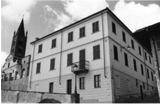
Figure 2. “Casa Capello” in Rivoli. On the background the bell tower of the Collegiata, on the foreground the breast wall that collapsed during the restoration works.
