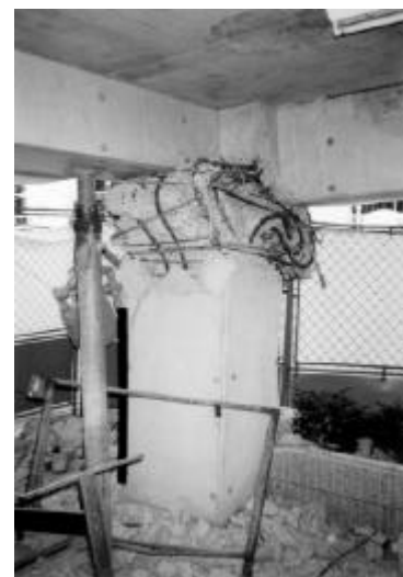
(c) Collapse caused by the reversed axial force due to overturning moment
