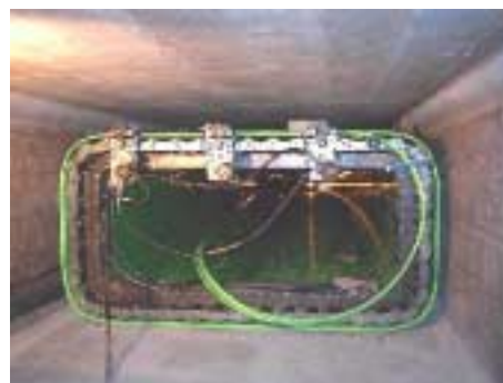
Figure 8. Installation of inner pipe with profile
