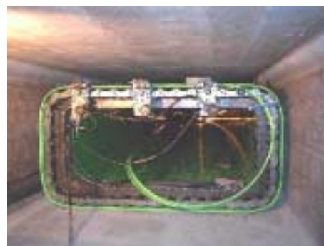
Figure 8. Installation of inner pipe with profile
