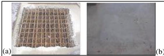
Figure 2. (a) Damaged concrete removed by a high-pressure water jet (hydro demolition) (b) repaired slab.
