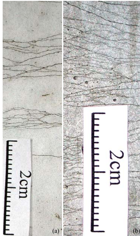
Figure 10. Multiple cracking pattern of Mix 3 (a) and Mix 4 (b)
