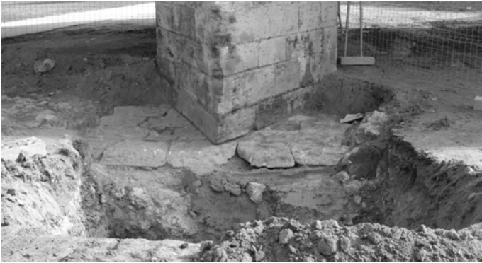
Figure 2. Foundations of the bridge.
