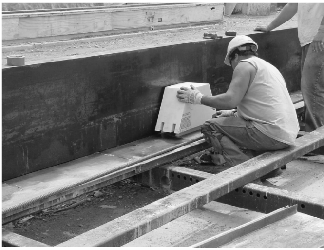
Figure 7. Blockouts for top strand beams.
