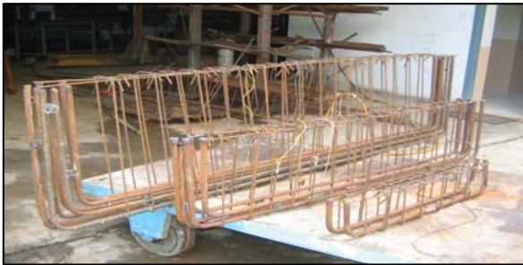
Figure 1. Typical reinforcement in RC Beam.
