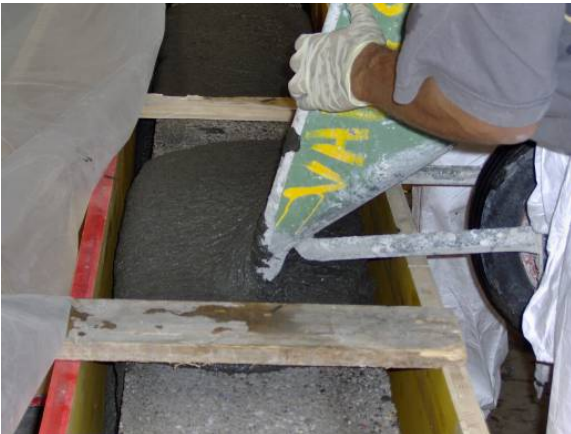
Figure 8. Casting of the HPFRCC layer.
