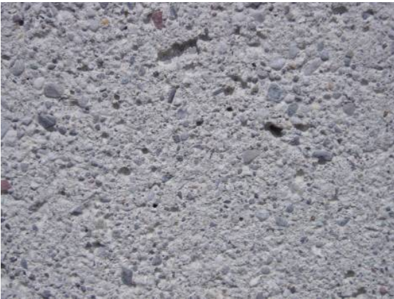
Figure 7. Sandblasting of the surfaces.
