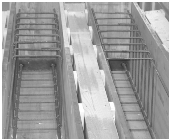
Figure 3: Detail of the steel rebars anchorage.
