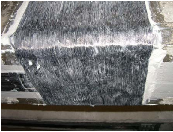
Figure 5. "U"-jacketing at one end of RC-N beam.
