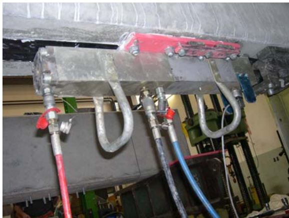
Figure 7. Hydraulic jack for pre-stressing CFRP laminate
