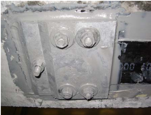
Figure 6. Steel bolted plate anchorages at both ends of RC-EA beam.
