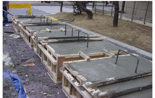
Figure 8. Concrete casted specimens.
