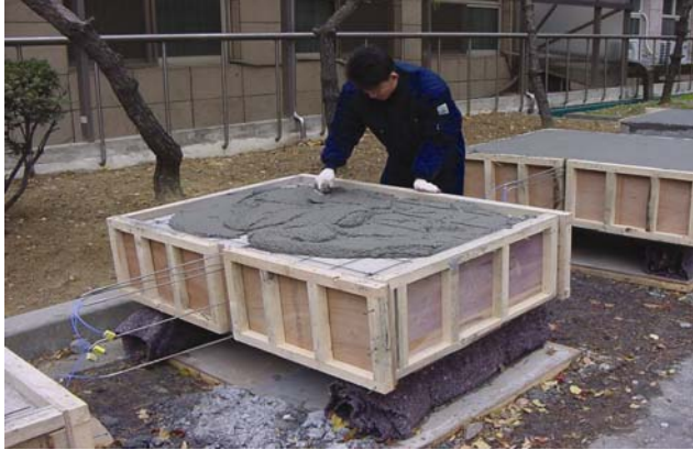
Figure 10. Coating the fire protection material by hand.
