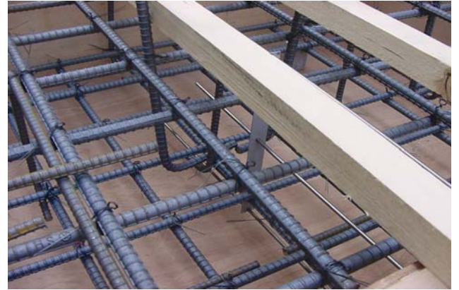
Figure 7. Installation of sheathed thermocouples.
