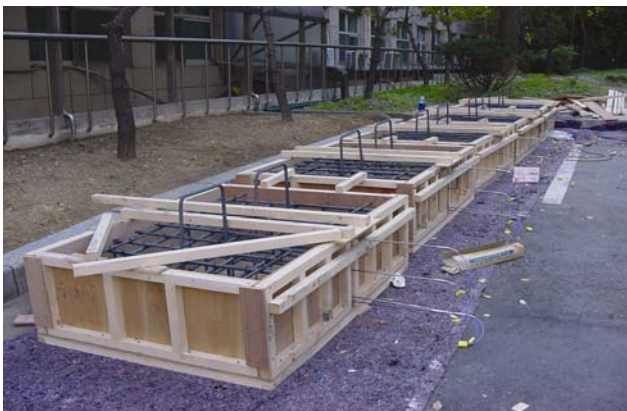
Figure 6. Formwork and reinforcing.
