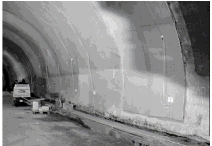
Figure 21. Arrangement of fire resistant concrete layer during the Virgolo tunnel test.
