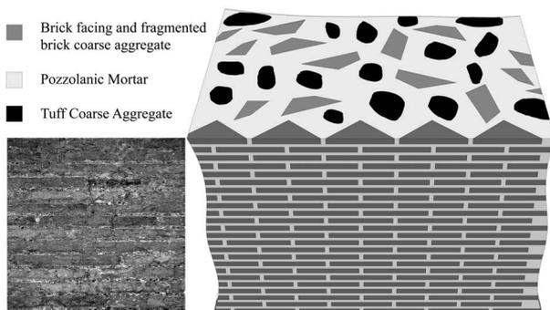
Figure 1. Photo of brick-faced concrete wall (bottom left) with schematic showing concrete nucleus. A typical facing brick is about 15cm wide.
