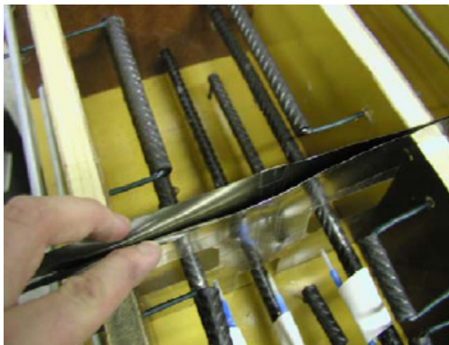
Figure 5. View into the prepared mould.
