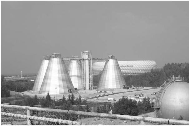
Figure 19. Newly-built digesters in the north of Munich.
