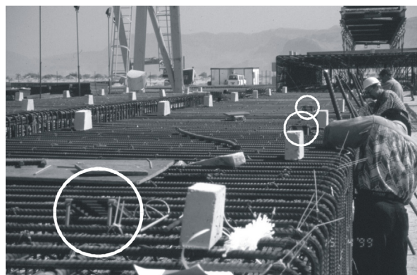
Figure 2. Sensors on the reinforcement belonging to a diaphragm wall, Al Sukhna, Suez Canal.
