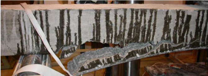
Figure 6. Concrete cover separation for the beam C13-M0-L6.
