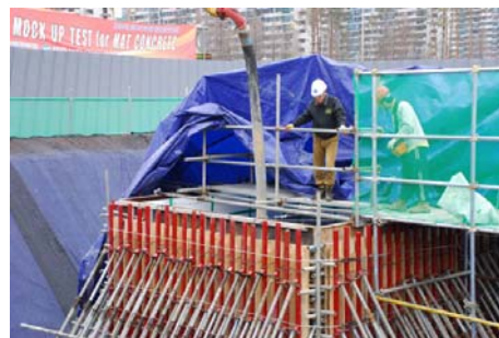
(b) Concrete placement
