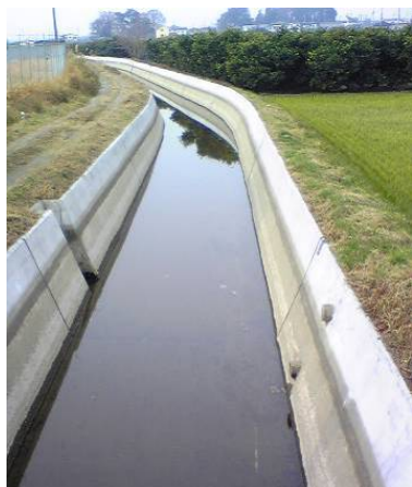
Figure 7. Waterway retrofitting application.
