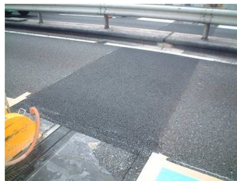
Figure 9. ECC joints in expressway
