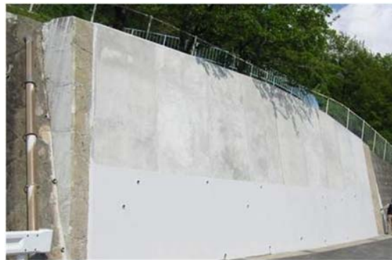
Figure 8. Retaining wall retrofitting application.
