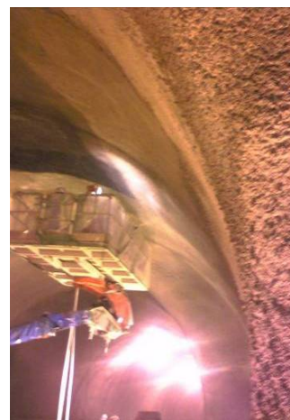
Figure 10. Tunnel lining with SHCC.
