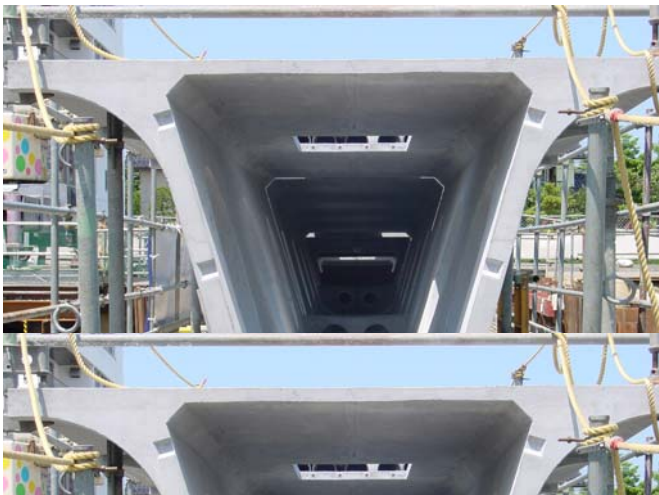
Photograph 2. Section of 1R pre-cast segment.
