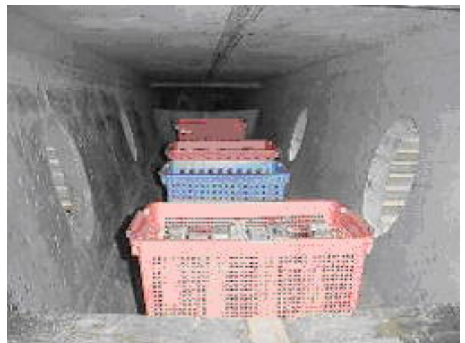
Photograph 4. Exposed specimens inside girder.
