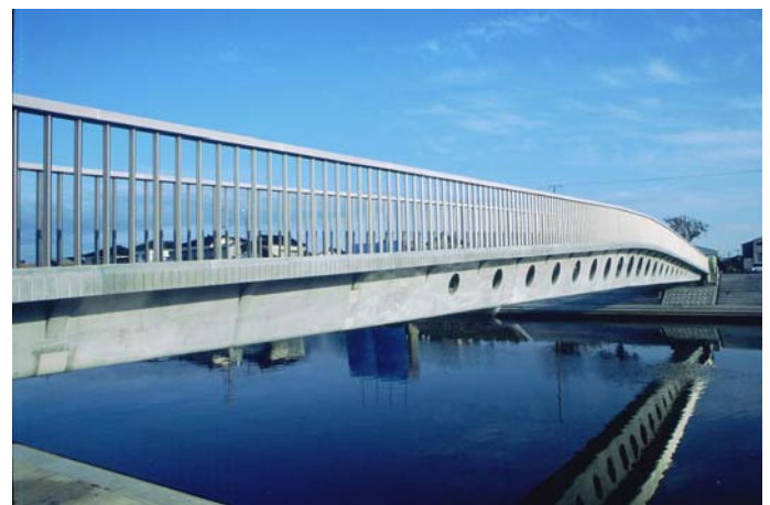
Photograph 1. Completion of Sakata-Mirai Footbridge.
