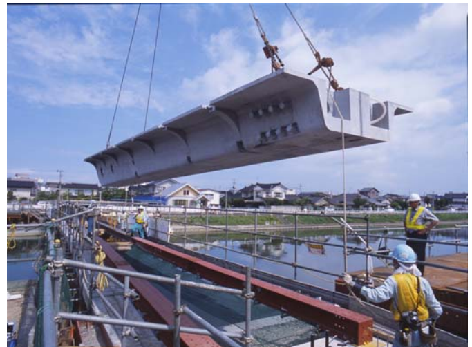
Photograph 3. Installation of 3L pre-cast segment.
