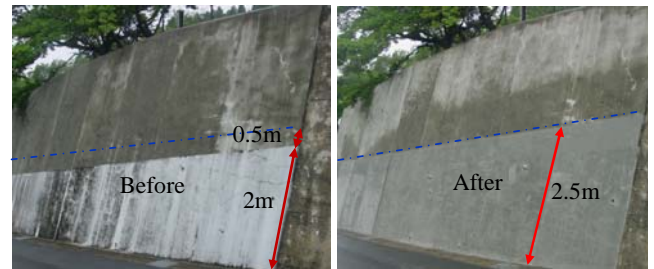
Figure 5. Appearances of wall before after water jet treatment.
