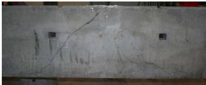
Figure 6. Crack pattern of RO80U2.
