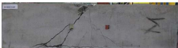
Figure 8. Crack pattern of RO80C4.
