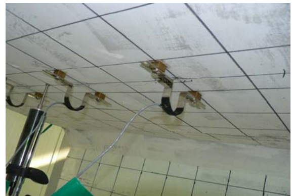
Photo 2. Closed view of Crack gauge and LVDTs.
