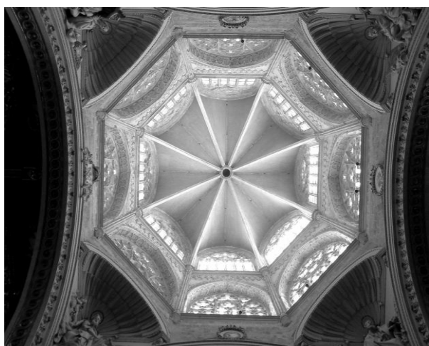
Figure 4: Image inside of the Cimborio
