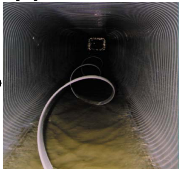
Figure 1: Sewer renovation by the SPR renovation method
