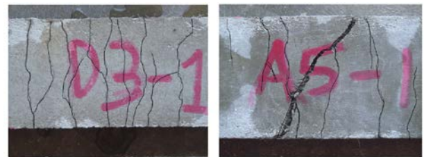
Figure. 7: Multiple Cracking Patterns in DFRCC (Left, PVA-1; right, ST+PVA-1)
