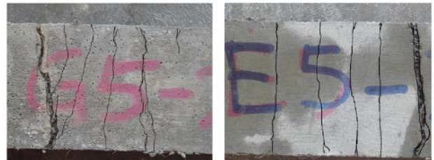
Figure. 8: Multiple Cracking Patterns in DFRGC (Left, PVA-1; right, ST+PVA-1)
