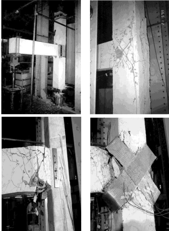
Figure 3: Joint failure of GRP rehabilitation ( Gobarah and Said, 2002 )
