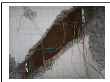
Figure 3: Removal of heavily damaged region of web.
