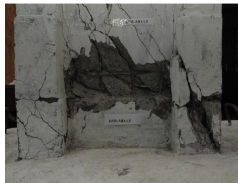
Figure 9: Spalling of concrete in web region and compression flange of RSW-MO-1.5.
