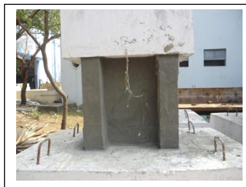
Figure 5: Shear wall after grouting and surface finishing.
