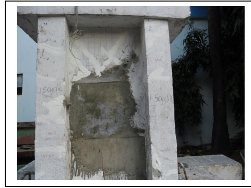
Figure 4: Replacement with new concrete.
