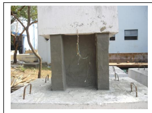
Figure 5: Shear wall after grouting and surface finishing.
