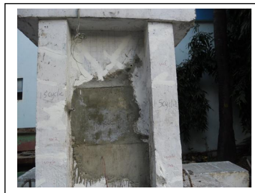
Figure 4: Replacement with new concrete.
