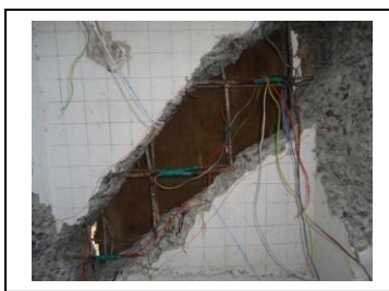
Figure 3: Removal of heavily damaged region of web.
