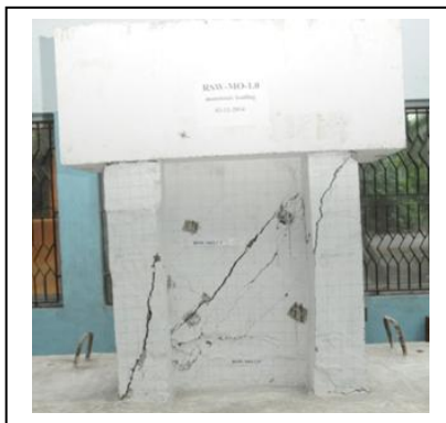
Figure 11: Final cracking pattern in shear wall RSW-MO-1.0.
