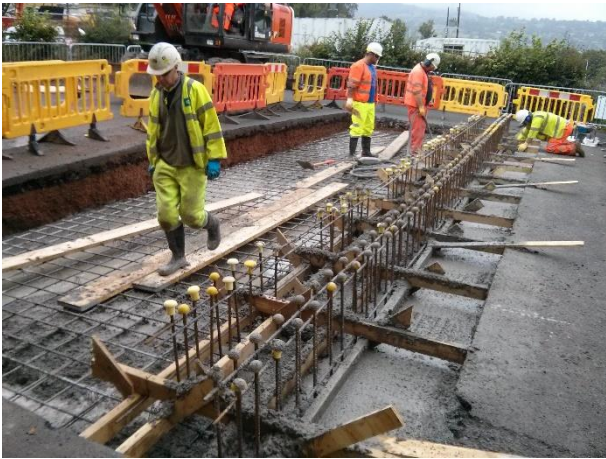
Figure 3: Casting of concrete base slab and kickers
