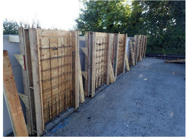
Figure 4: Formwork and reinforcement setup for trial panels
