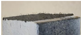
(a) Concrete PA
