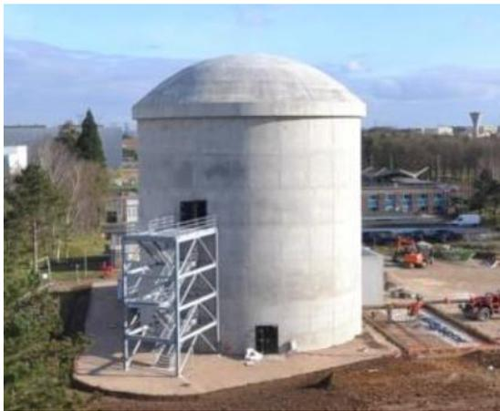
**Figure 1:** Nuclear reactor building VeRCoRs mock-up [12]
