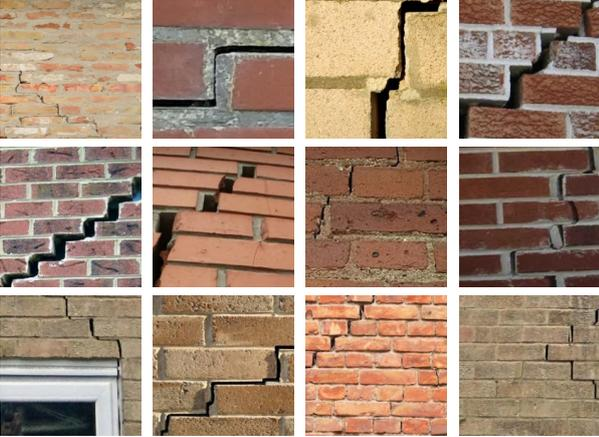
Figure 3: Examples of cracks in bonded masonry structures [5].
