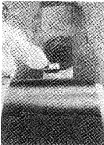
Photo 3 Gluing CF sheet on chimney in the vertical direction
