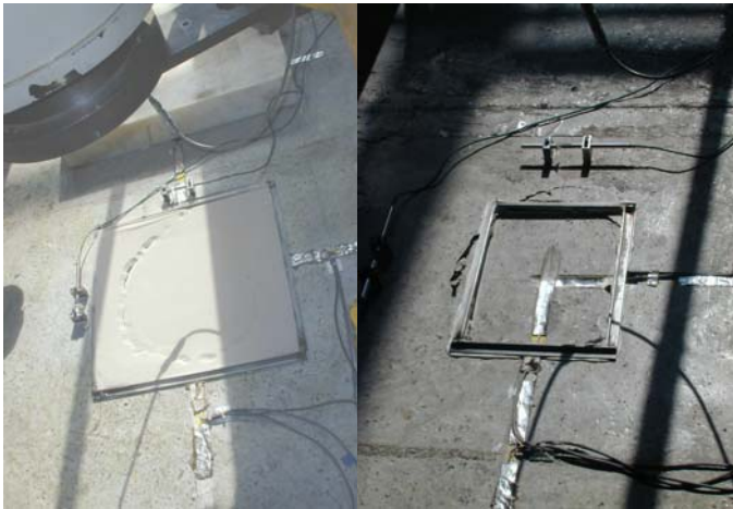
Figure 17. left) Zone N2N3 after failure. Failure on top is concentrated around the reduced loading plate even with sand cushion over the 0.4 m-square surface (configuration 3). Right) Zone N3N4 after failure (configuration 4).
