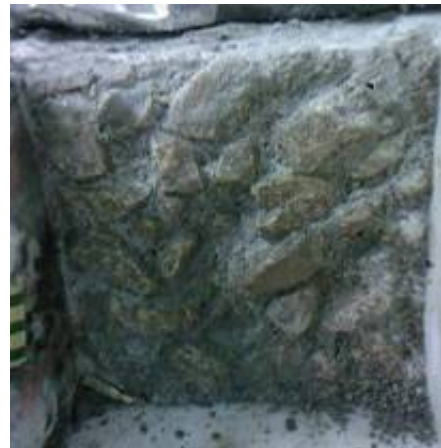
Figure 17. Surface state for the construction joints.
