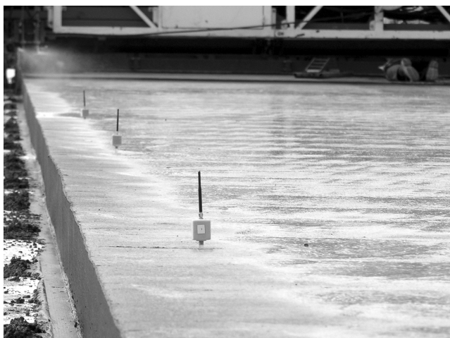
Figure 9. Wireless capillary pressure sensors on a road construction site.
