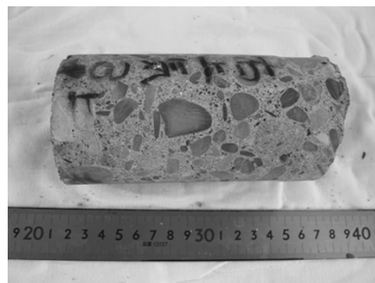
Figure 6. Type C sample (non-cracked concrete).
