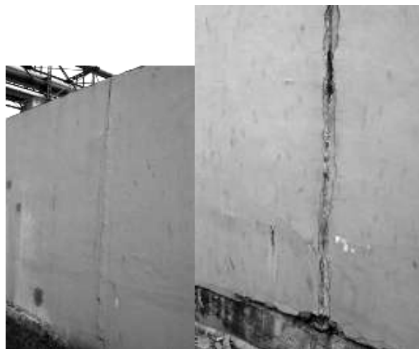
Figure 14a and 14b. Vertical dilatation joint were covered with repair mortar (14a). Typical result of thus rehabilitation is shown on the right (14b).
