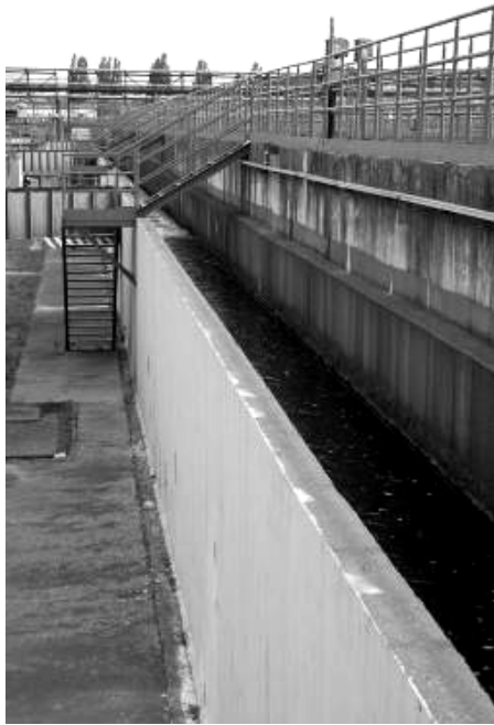
Figure 1. Reinforced concrete discharge conduit from final setting tanks.
