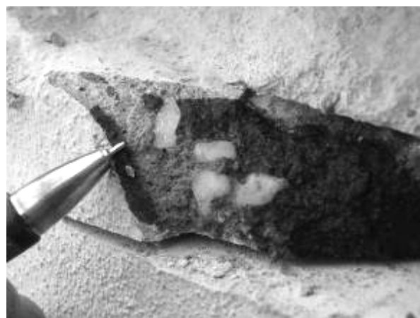
Figure 13. Repair materials were applied on carbonated layer of concrete.
