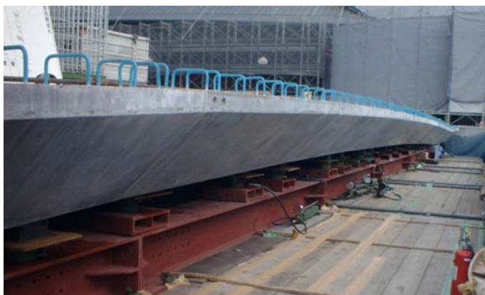
Photograph 3. Dry joint for pre-cast segment.
