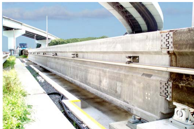
Photograph 4. Completion of 40m long monorail girder.
