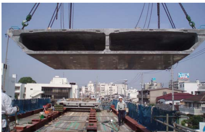
Photograph 2. Erection of pre-cast segment.
