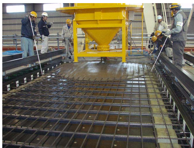
Photograph 12. Casting UFC to mould.
