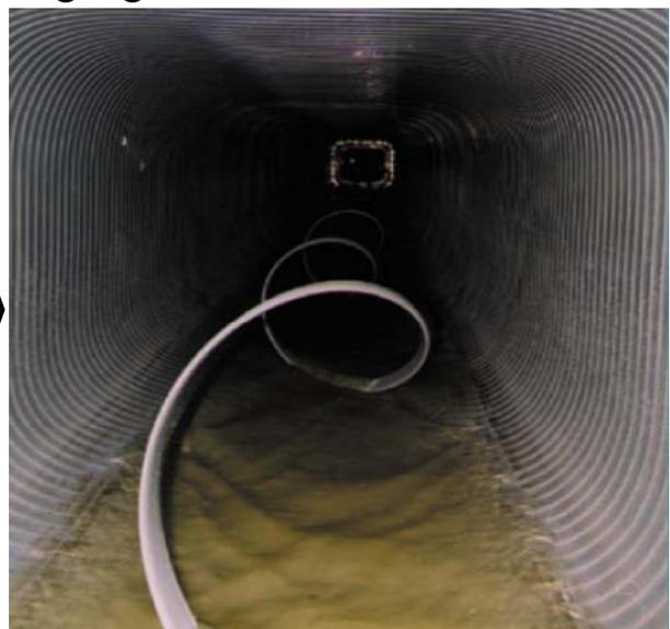
**Figure 1:** Sewer renovation by the SPR renovation method
