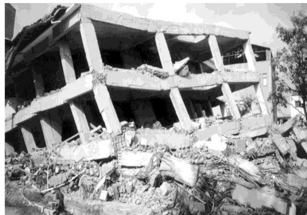
**Figure 1:** Beam-column joint shear failure in RC buildings [1].
